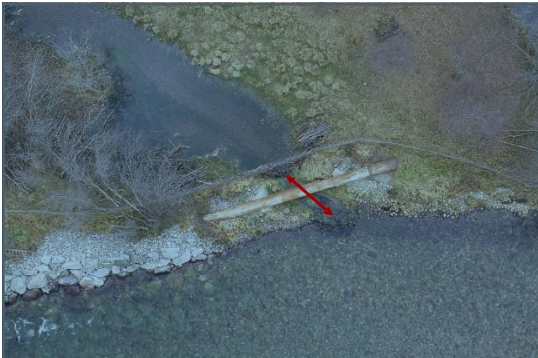
Figure 9 Adjustments to the outlet
